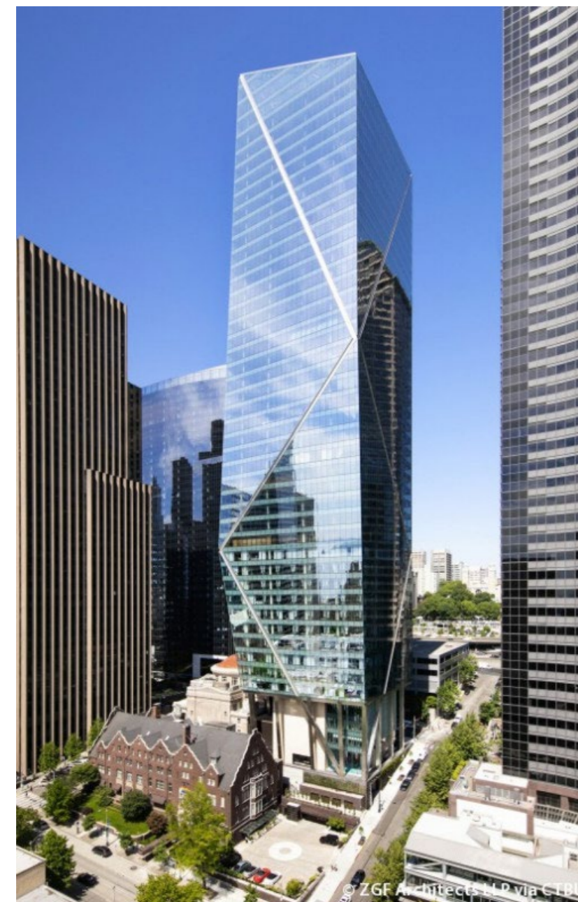
Seattle's F5 Tower pictured above
